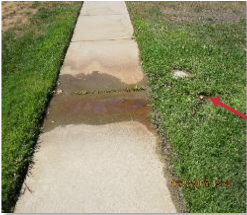
Broken/ leaking sprinkler heads
