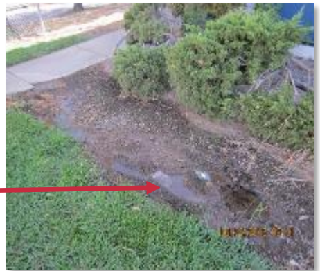
Broken/ leaking sprinkler heads
