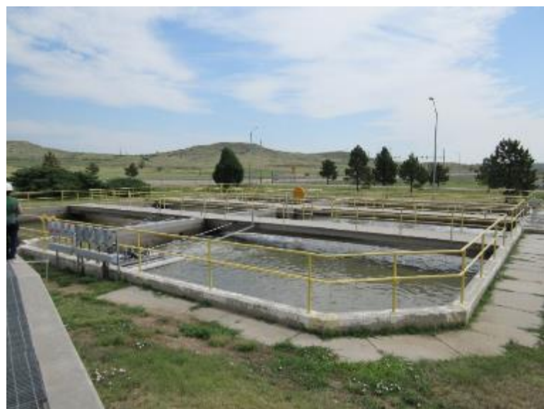
Fort Carson Reclaimed Wastewater
